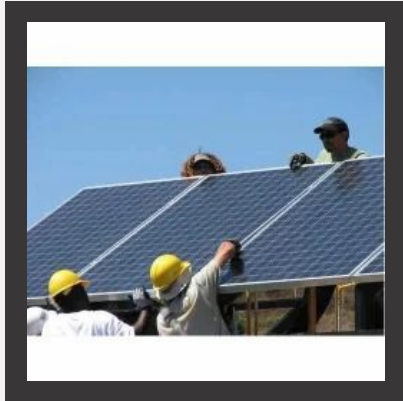
Solar Lighting System
