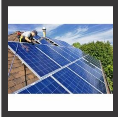
Solar Panel Installation
