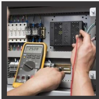
Ups Maintenance Service
